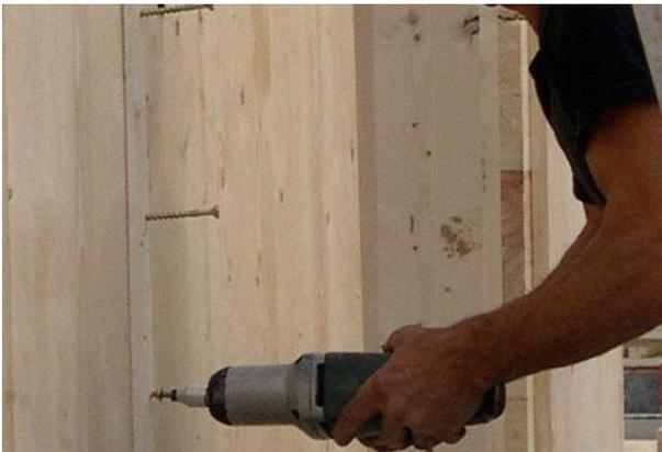
**Figure 9:** Screwing in vertical position
