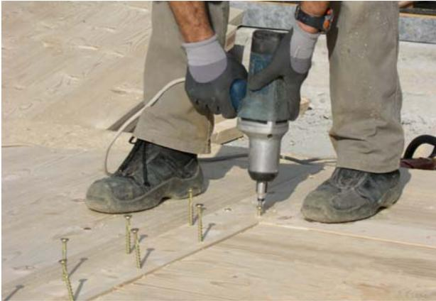
**Figure 8:** Screwing in horizontal position
